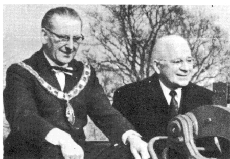
Mr. Herbert Armstrong (right) astride bulldozer at Bricket Wood, England.
